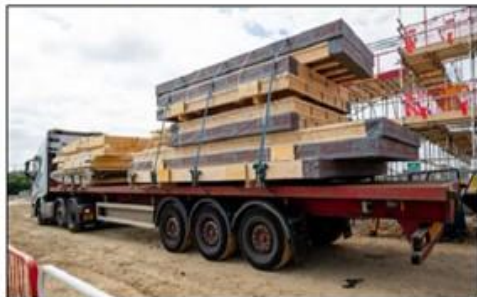
7 – Delivery to site
