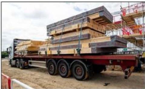
7 – Delivery to site
